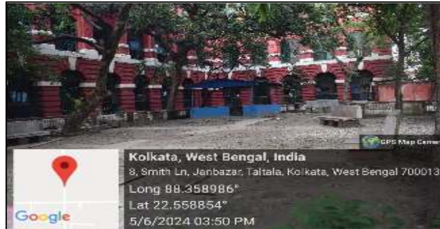
BUILDING OF BAKER GOVT. HOSTEL
