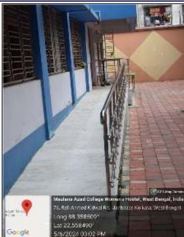
RAMP AND RAIL FOR DIVYANGJAN INMATES
