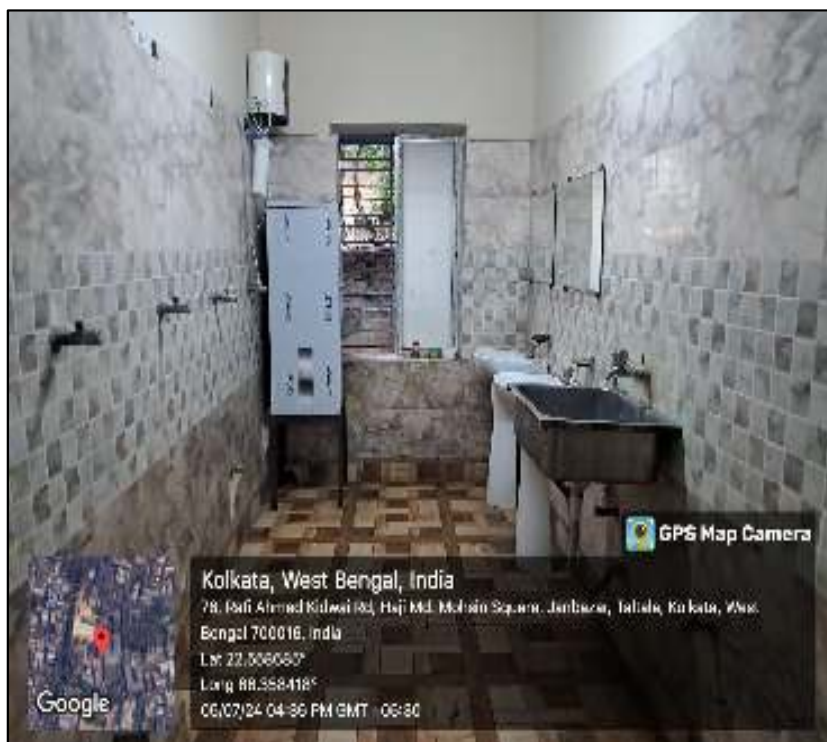
WELL MAINTAINED WASH BASINS
